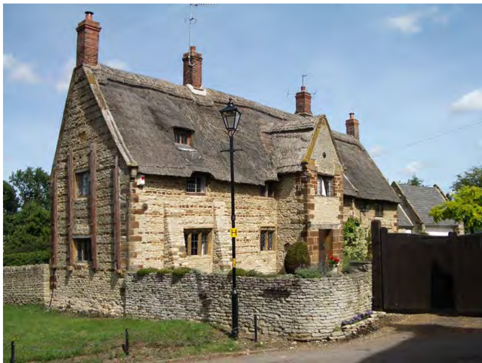
Alternate limestone with narrow bands of ironstone is an attractive feature of a number of buildings, as seen here on the 17 th century Manor House (listed grade II*)
